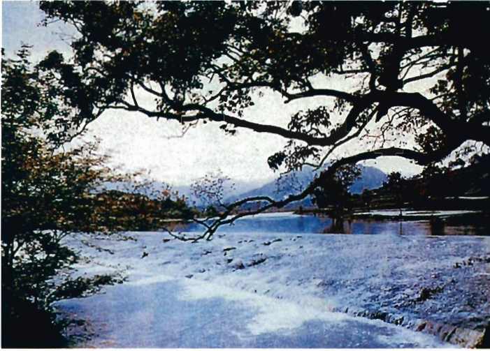
LEFT (135) A spillway of the world's oldest contour transport canal, the Ling Ch'u, or Magic Canal, which connects the River Li and the River Hsiang and was constructed in the third century BC (though since restored and improved).
