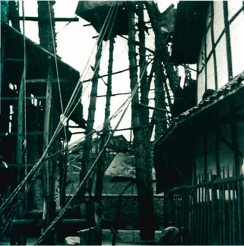
LEFT (31) A photograph taken by Cecil Beaton during the Second World War, showing a traditional Chinese deep-drilling derrick over the well head of a brine and/or natural gas well.
